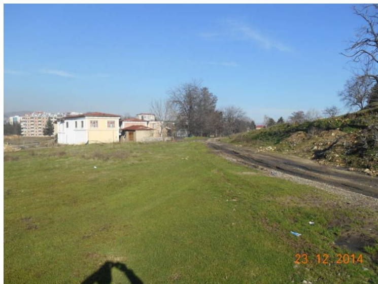
Figure 16 Current condition of the street SrU 4 in ARM district 2 Source: CeProSARD's archive
