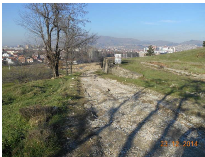
Figure 18 Current condition of the street StU 12 in ARM district 2 Source: CeProSARD’s archive
